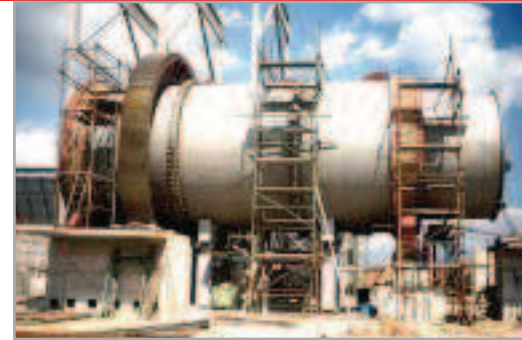
Assembly of a raw mill Ø 5.4 x 11 m with pre-drying chamber
