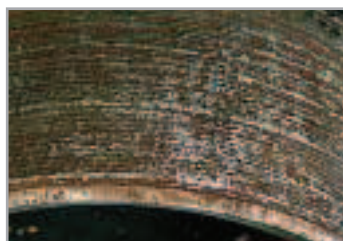
Hard facing on the runner casing
